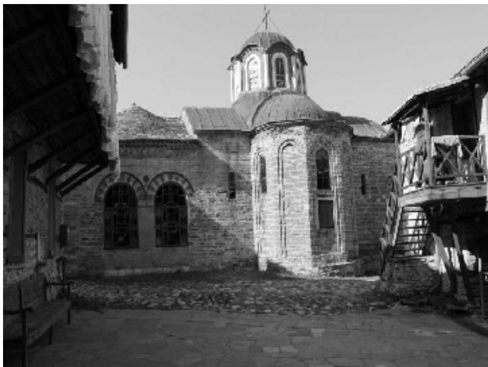
Photo 1. (It shows the southern side of the church) A. Palushi
