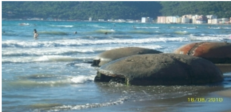
Fig.2. View from the coast of Kune-Vaini, where the bunkers remaining in water show clearly the powerful erosion over the last 30 years.
