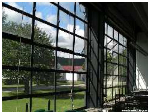
Penetration of light in Fagus factory's building
